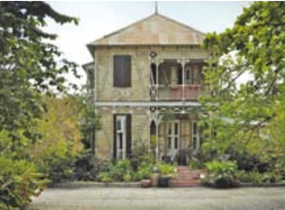
'Gingerbread' house in Port-au-Prince. © Randolph Langenbach
