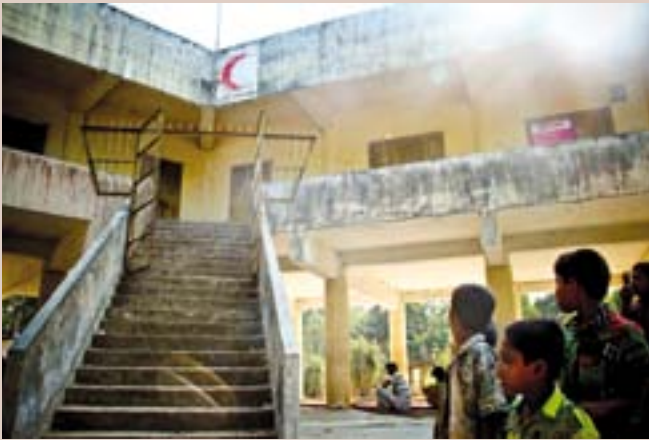
Shelter built by the Bangladesh Red Crescent Society in Cox’s Bazar where BRAC has set up a primary school. ©Himadri Ahsan/BDRCS.
