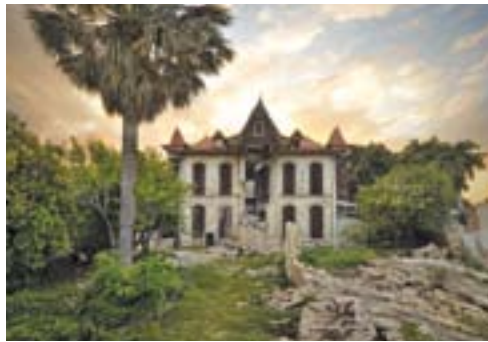
The Villa Castel Fleuri, which was constructed with walls of brick and rubble stone, was still standing after the 2010 Haiti earthquake. © Randolph Langenbach
