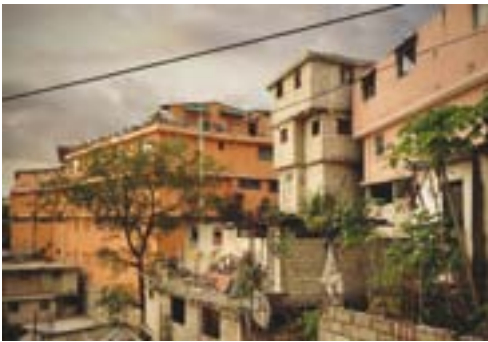
Non-engineered concrete block and slab houses in Jalousie informal settlement, Petionville, many of which survived the 2010 earthquake. © Randolph Langenbach
